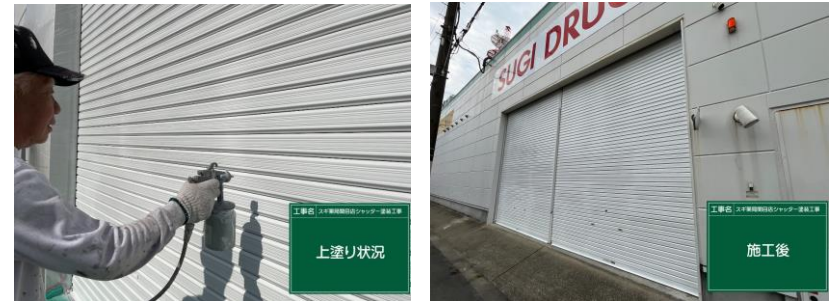
Heat-shielding coating applied to a shutter at a drugstore in Osaka – May 2025
