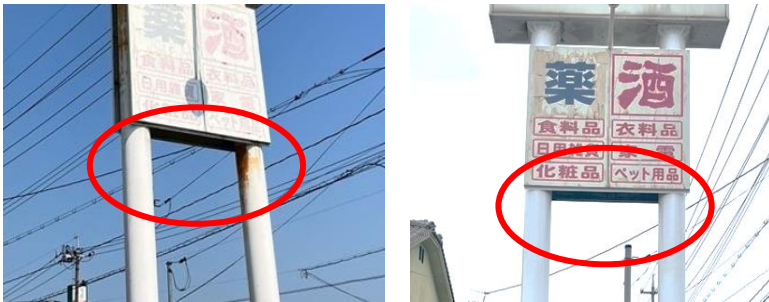
In June 2025, a sign pole at a drugstore in Hiroshima Prefecture was coated for rust prevention.
