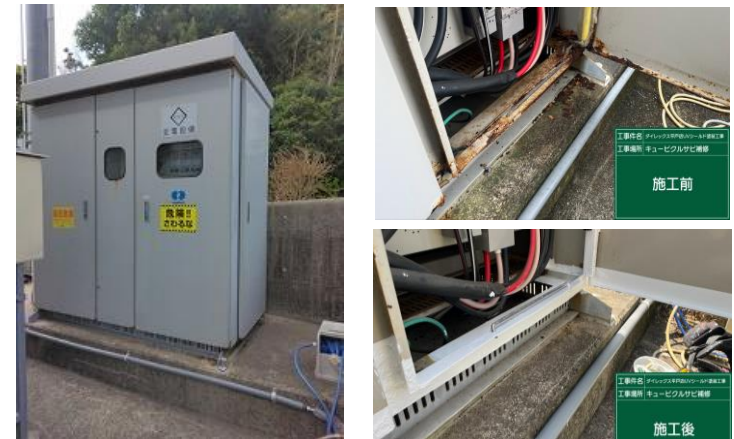
Rust prevention coating inside a cubicle at a seaside supermarket in Nagasaki – June 2025
